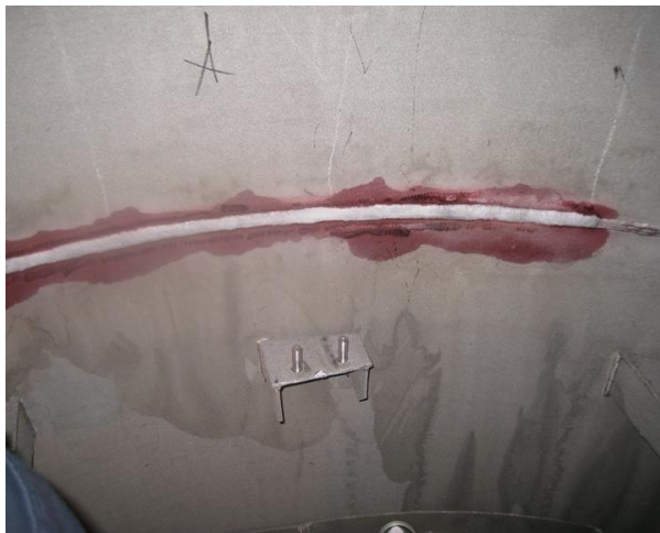
Figs.11 & 12: (Repaired area) &( Repaired Weld)
